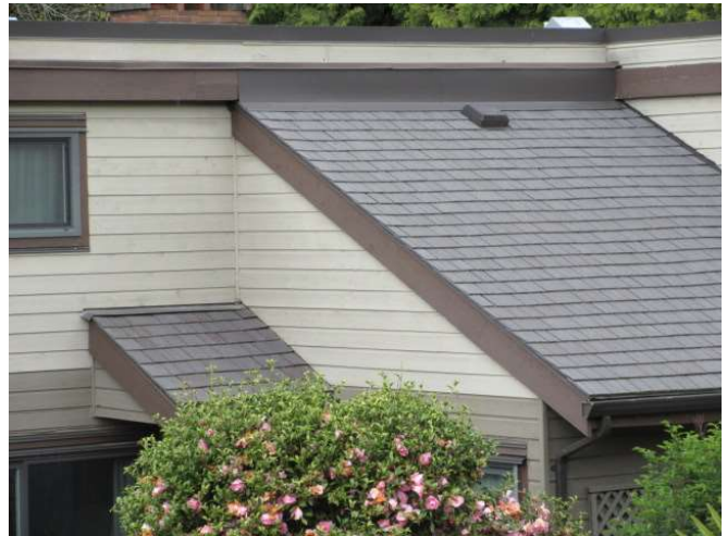
Photo 11: Sloped roofs with Enviroshake shingles at building 15.
