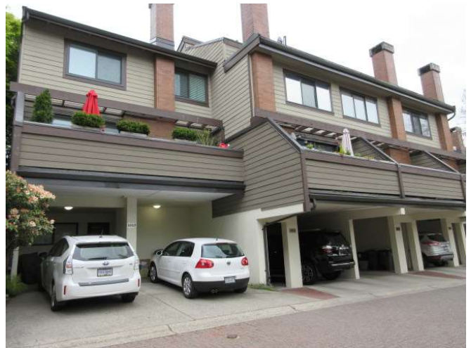
Photo 4: Typical balconies at building 1.
