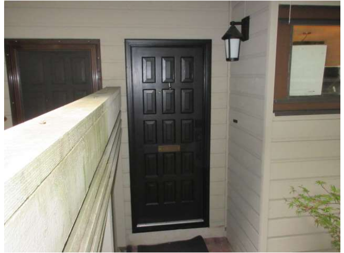
Photo 8: Typical exterior entrance doors.
