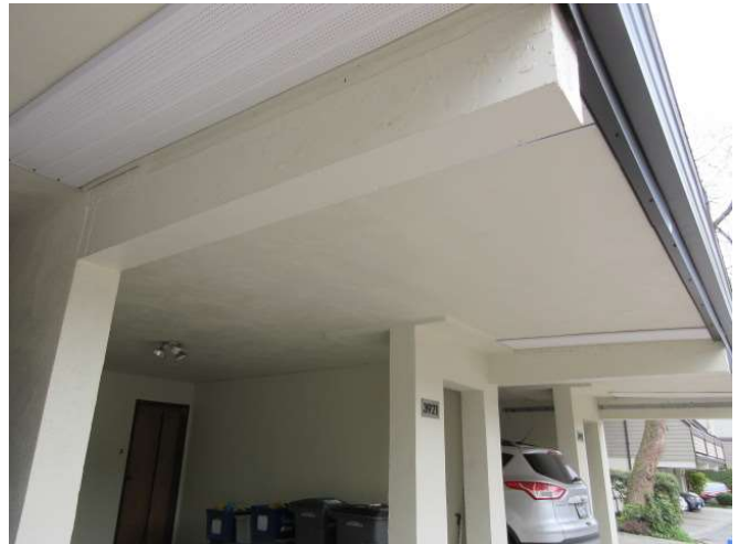
Photo 1: Typical concrete framed parking areas at Buildings 1, 3, 5 and 7.
