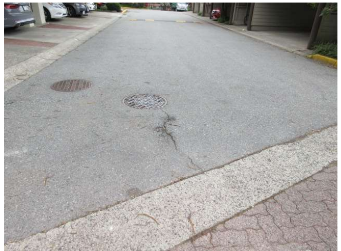
Photo 19: Typical sanitary sewer manhole covers.
