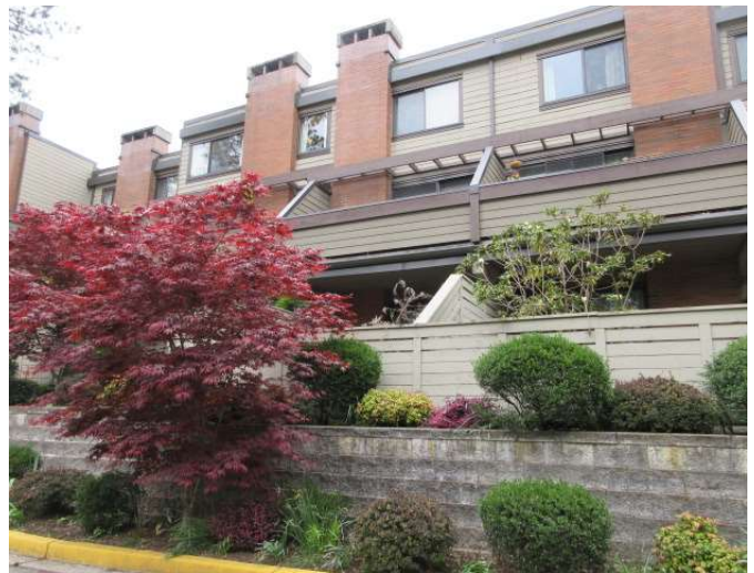
Figure 2: Typical newer retaining wall, patios with fences and balconies above.
