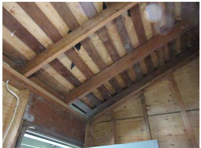
Photo 12: Underside of roof in pool house with original wood strapping and plywood sheathing over top.
