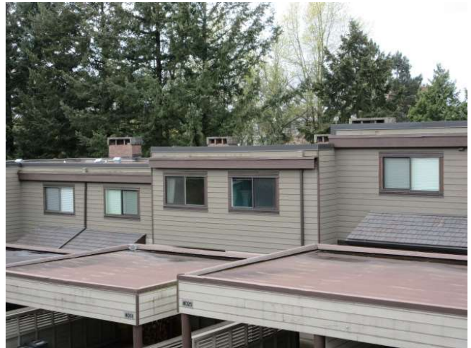
Photo 9: Typical flat roofs over the buildings and carports.
