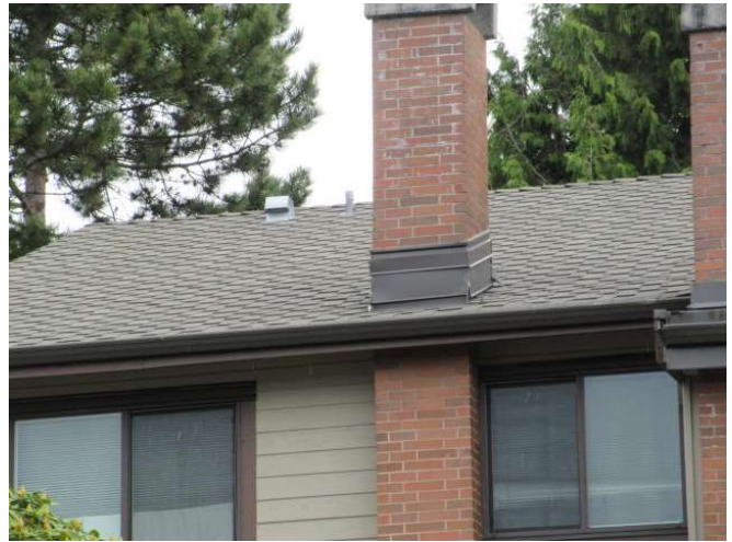
Photo 10: Typical sloped roof with asphalt shingles.
