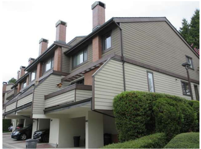
Photo 5: Typical exterior walls.
