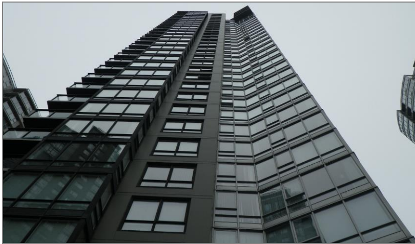
Figure 2.1 Elevation Photo South elevation of the building.
