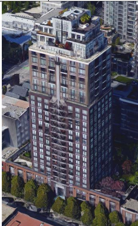
Figure 2.2 Aerial photograph of Domus (© 2018 Google Maps).
