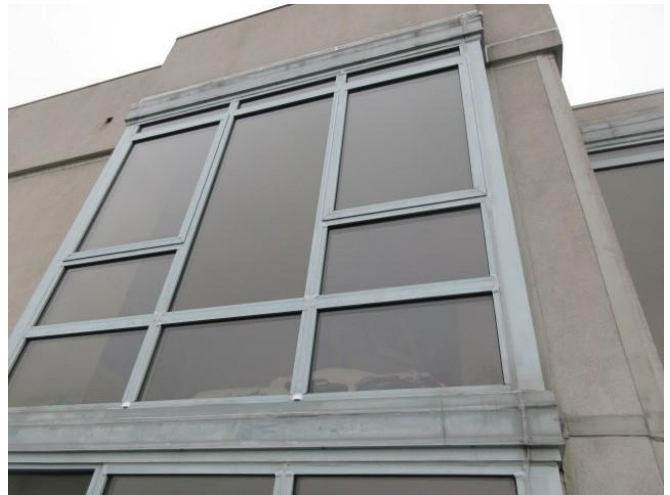
Photo 6: Typical window wall.
