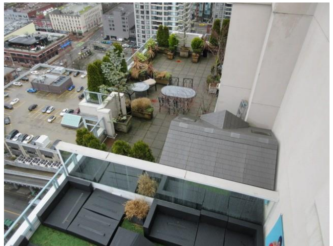
Photo 9: 30th floor roof decks.
