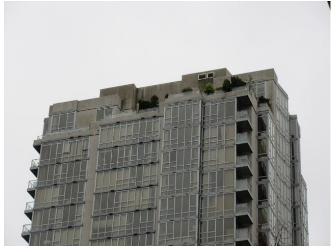
Photo 2: Typical balconies at corners of the building.
