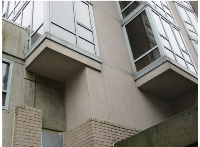
Photo 5: Typical exterior walls.
