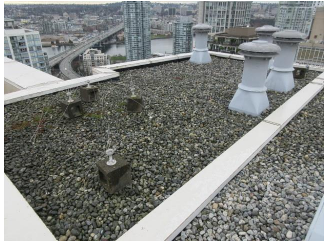
Photo 8: Mechanical penthouse roof.
