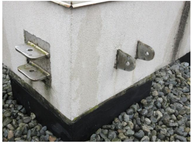
Photo 3: Typical roof anchors.
