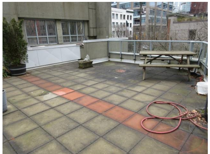
Photo 10: 2nd floor roof deck.
