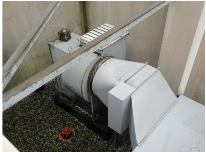
Photo 17: Smoke exhaust fan.
