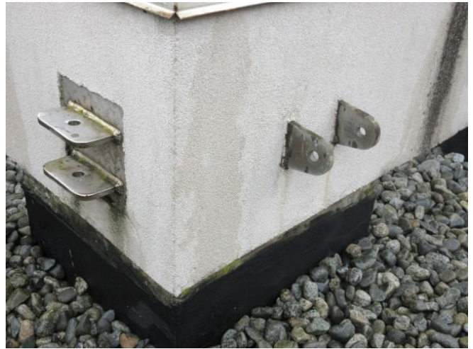
Photo 3: Typical roof anchors.
