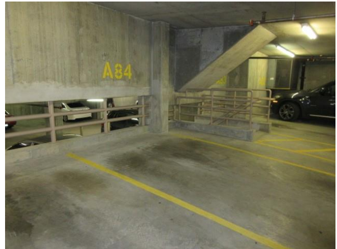
Photo 4: Typical parking garage.
