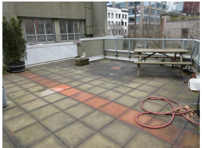
Photo 10: 2nd floor roof deck.
