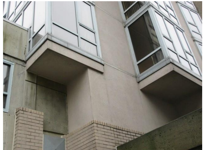
Photo 5: Typical exterior walls.
