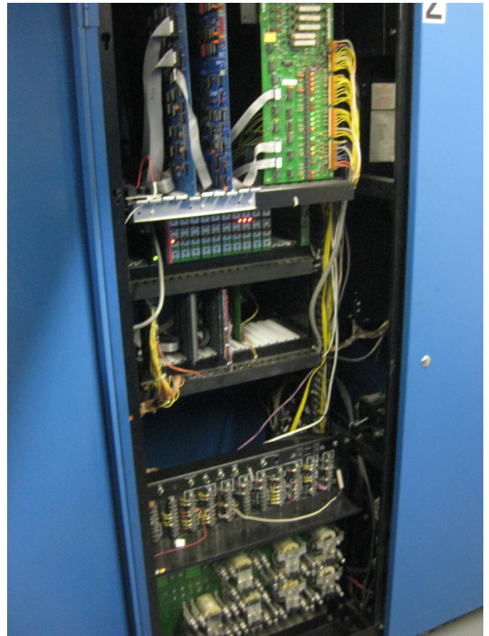
Figure 4 – Elevator Controller
