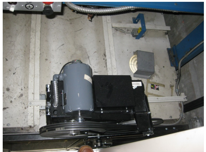
Figure 8 – Door Operator
