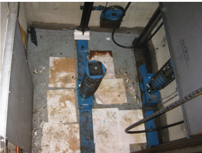
Figure 6 – Elevator Pit – Car 1 (note absorbent pads)
