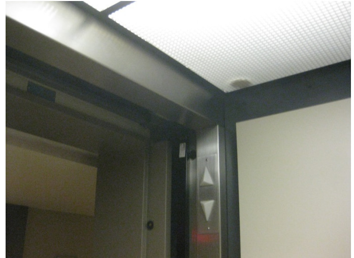
Figure 11 – Interior Finishes and Fixtures
