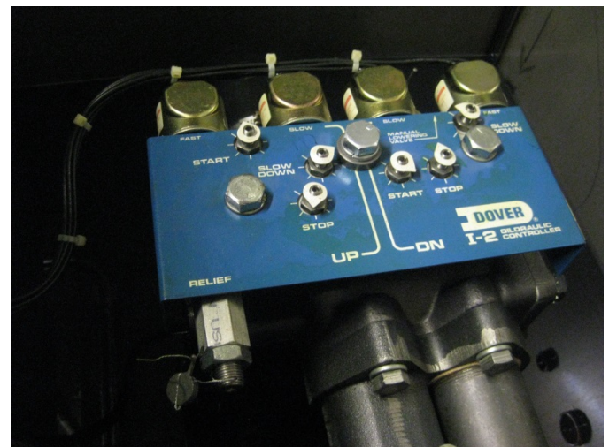
Figure 12 – Hydraulic Valve
