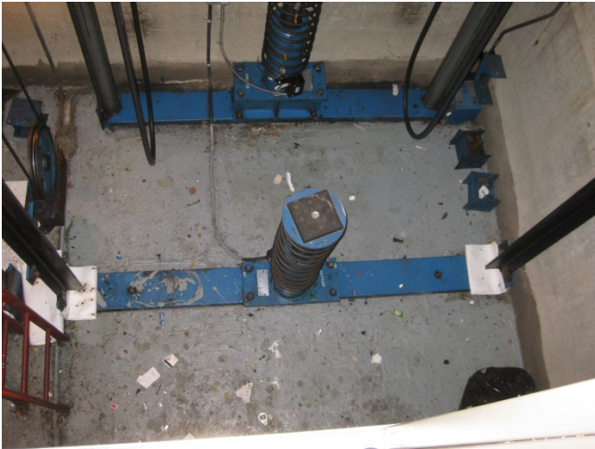
Figure 5 – Elevator Pit – Car 2
