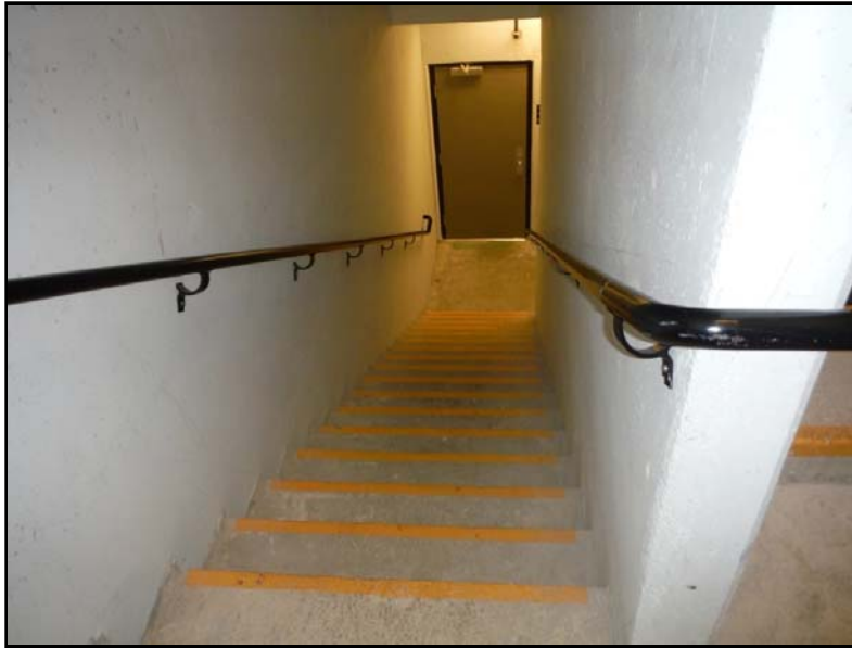
Photo No. 19: Typical stairwell
