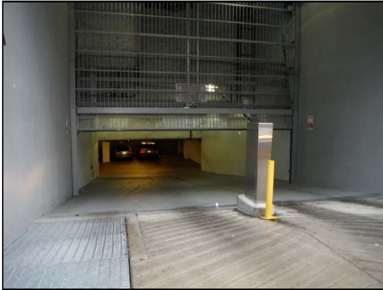
Photo No. 3: Garage entrance
