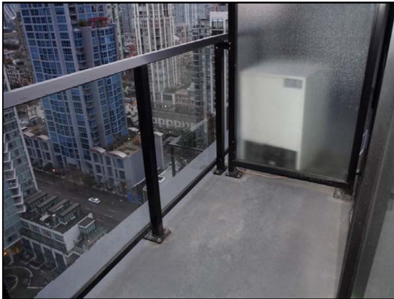
Photo No. 5: Typical balcony
