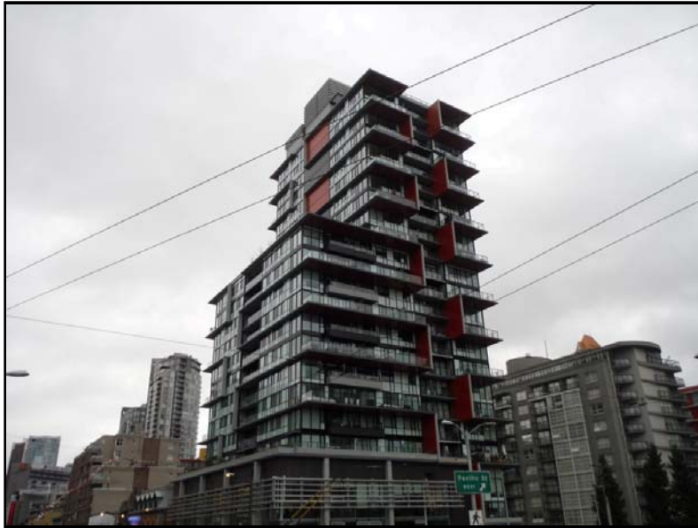
Photo No. 1: West elevation
