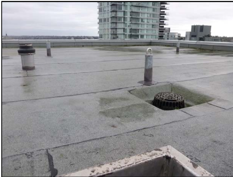
Photo No. 7: Typical flat roof area
