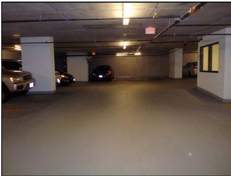
Photo No. 4: Typical garage area
