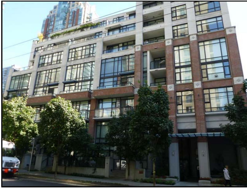
Photo No. 1: West elevation
