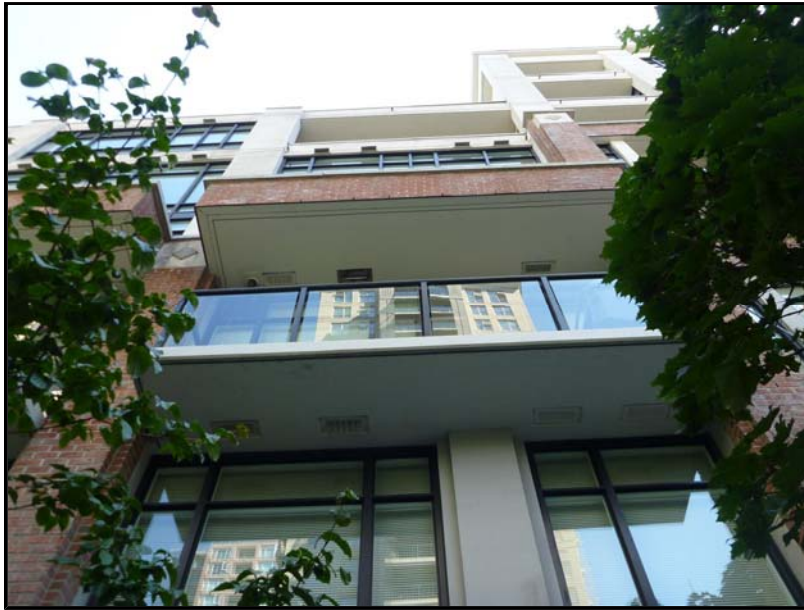
Photo No. 3: Balconies
