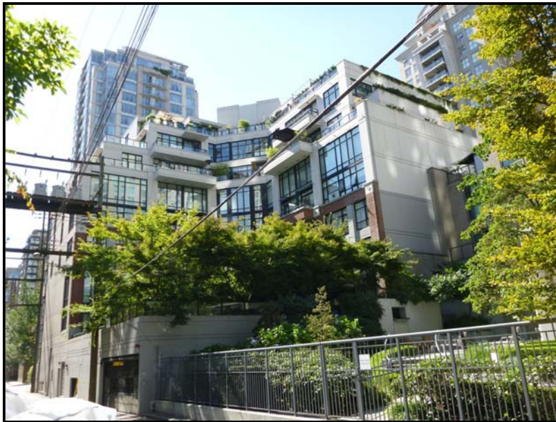
Photo No. 2: North and east elevations and courtyard
